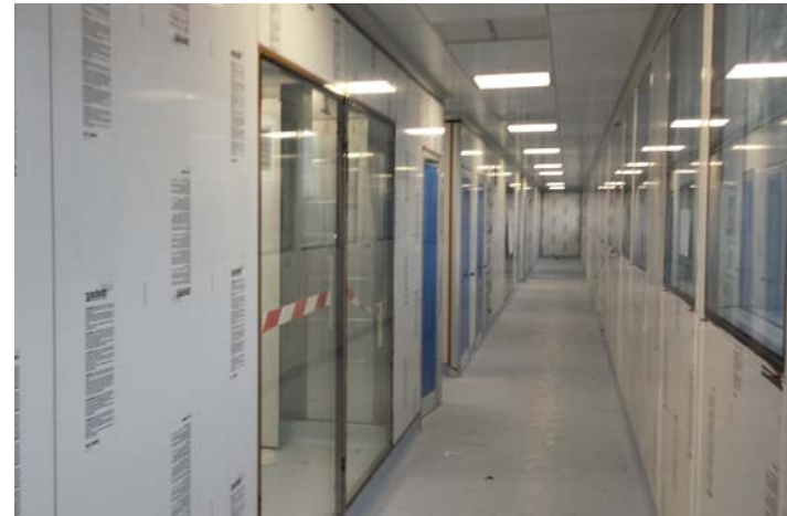
Grade C Corridors – walls, windows and false ceiling in sealing step
